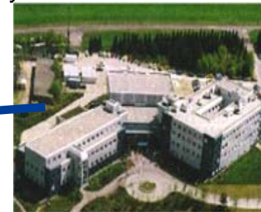
GSOC Control Center
