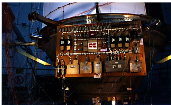
Figure 2: Instrumentation Platform of MAQSATH with power, amplifiers and telemetry
